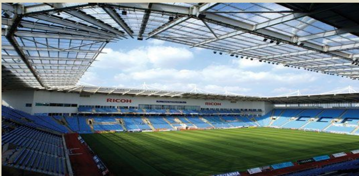
South, West and North Stands
